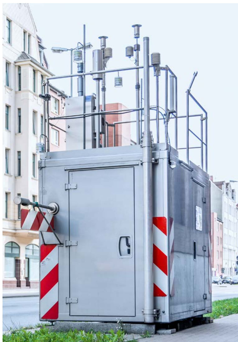
Measuring station for immission monitoring
